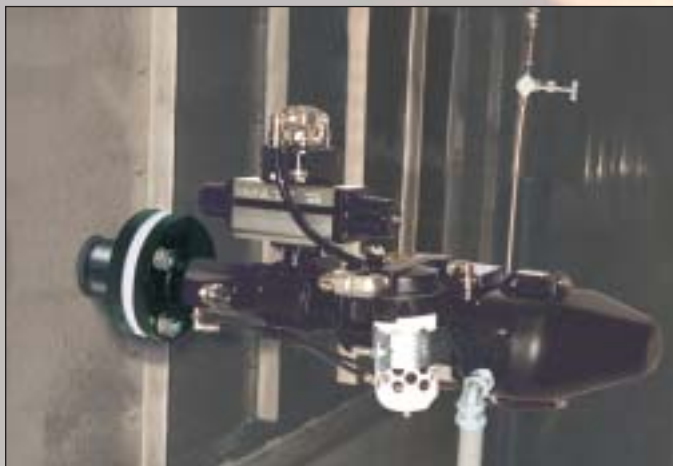
Infra-View ® Boiler / Furnace Thermometer mounted on boiler with optional air actuated Infra-View ® Valve designed to open with air purge and spring to close to protect sensor on plant air loss.
